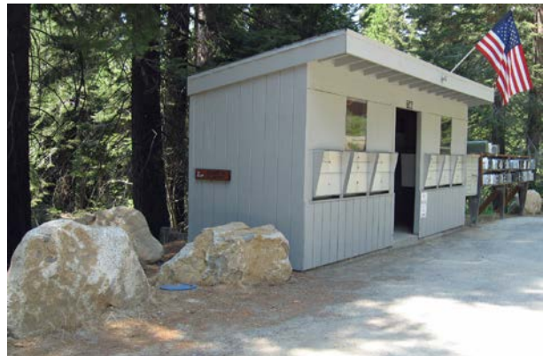
Newly painted mailbox shed with protective boulders
